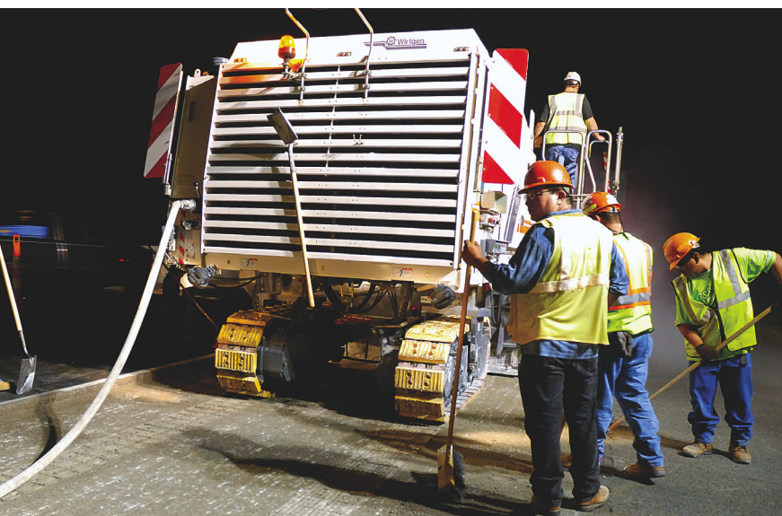
Lane Construction mills concrete lanes at night in reconstructing I40. Photo: Wirtgen
